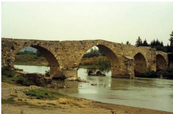
The multi-span Köprüpazar Bridge, 13 th c.
